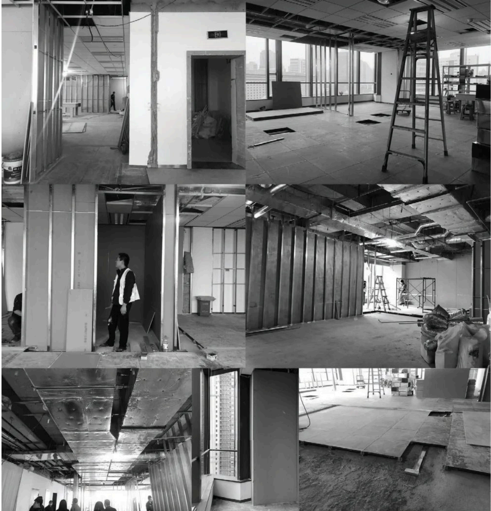
On-Site Construction Photos
